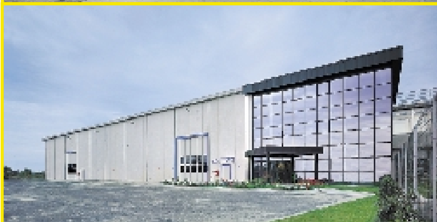
Factory and offices: CARONNO PLLA - VA Factory: QUARTO D'ALTINO - VE
